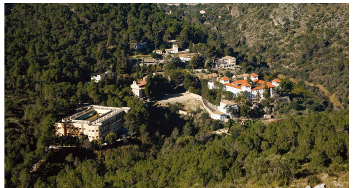
The Fontilles sanatorium is located in a valley that keeps the buildings hidden from neighboring towns while also offering a view of the sea.
